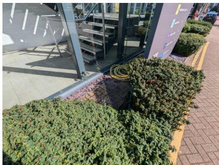
PHOTOGRAPH 5 LOCATION OF EXISTING LANDLORD CHAMBER IN LANDSCAPED AREA ADJACENT TO PARK SIGN
