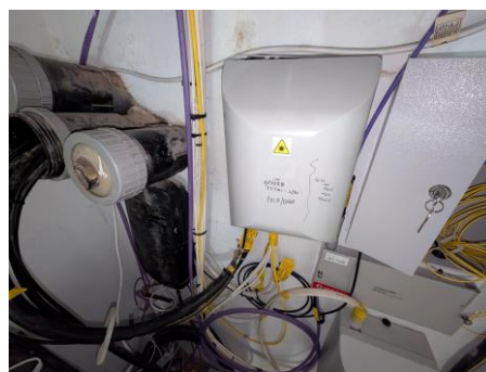
PHOTOGRAPH 11 EXISITNG BT FIBRE BFP
