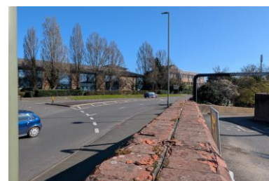
VIEW LOOKING EAST ALONG THE CAUSEWAY
