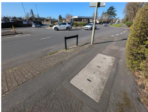
PHOTOGRAPH 1 EXISTING BT CHAMBER IN FOOTWAY ON THE CAUSEWAY NEAR TO ESTATE ACCESS ROAD
