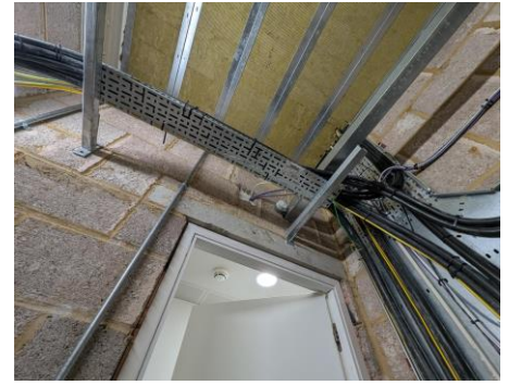
PHOTOGRAPH 24 TYPICAL VIEW OF ACCESS TO CEILINGS
