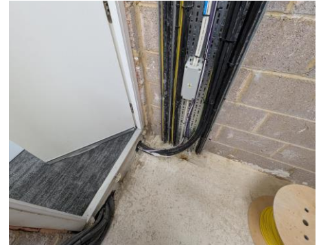
PHOTOGRAPH 27 TYPICAL VIEW OF ACCESS TO RAISED FLOOR
